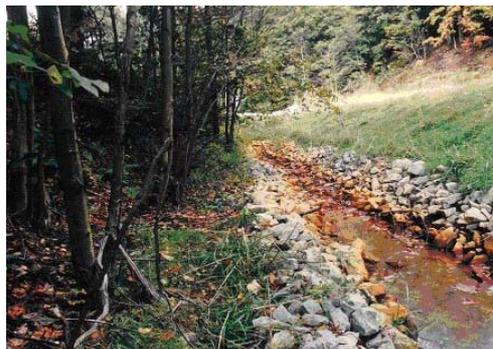
Open Limestone Drain showing a build up of iron precipitates (brown) coating limestone fragments.
