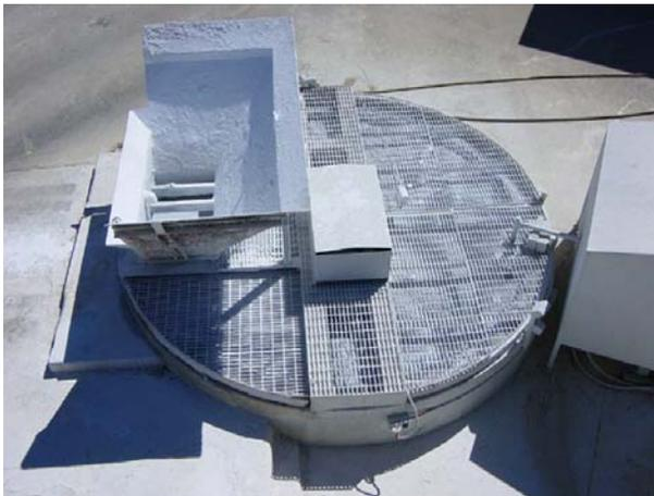
Figure 5. Below ground hydrated lime storage, mixing and dosing system.
