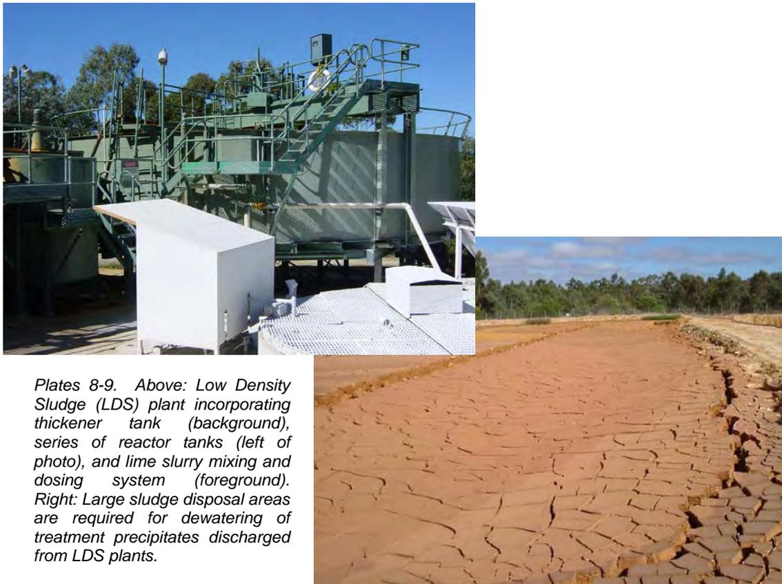
*Plates 8-9. Above: Low Density Sludge (LDS) plant incorporating thickener tank (background), series of reactor tanks (left of photo), and lime slurry mixing and dosing system (foreground). Right: Large sludge disposal areas are required for dewatering of treatment precipitates discharged from LDS plants.*
