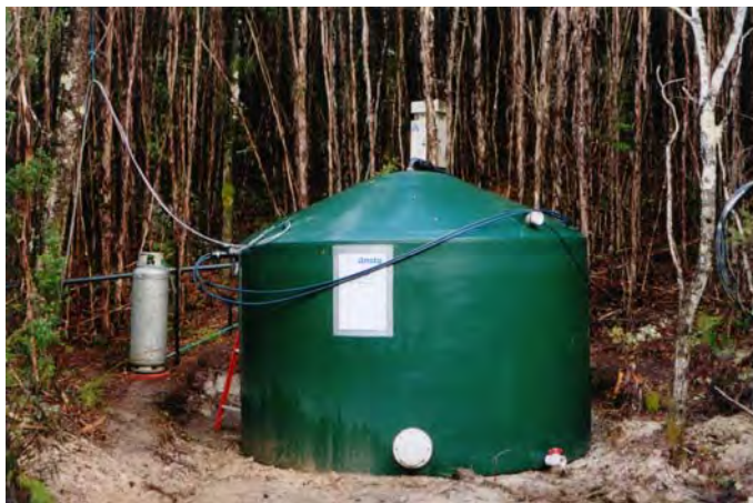
Plates 4-5. Gas Redox and Displacement System (GaRDS) for prevention of AMD formation in an underground mine. Left: Bioreactor used to generate CO 2 and CH 4 gases, which displace oxygen from the mine. Right: Installation of low permeability wall and drainage system at the main adit opening.
