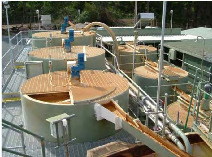
Plate 10. High Density Sludge (HDS) plant used for the continuous treatment of AMD from a decommissioned mine site. Key sources of AMD at the site include pit wall rock and benches, waste rock dumps and a tailings storage facility.
