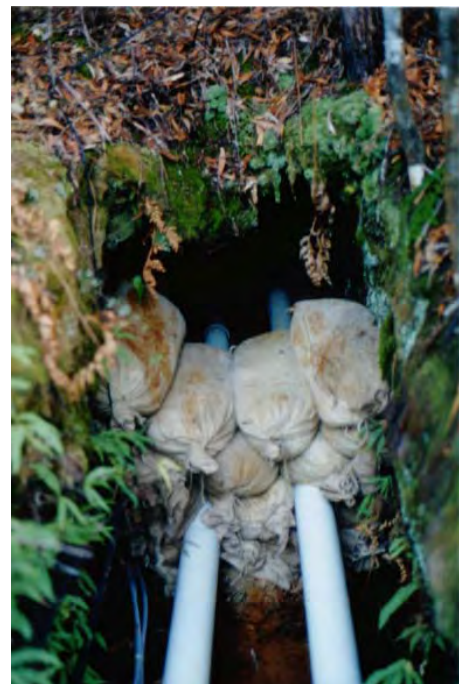
Plates 4-5. Gas Redox and Displacement System (GaRDS) for prevention of AMD formation in an underground mine. Left: Bioreactor used to generate CO 2 and CH 4 gases, which displace oxygen from the mine. Right: Installation of low permeability wall and drainage system at the main adit opening.
