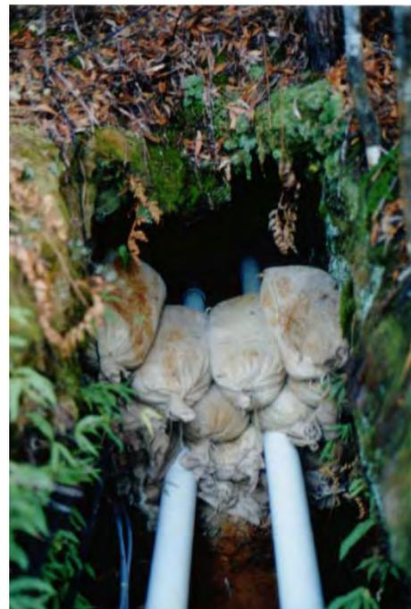
*Plates 4-5. Gas Redox and Displacement System (GaRDS) for prevention of AMD formation in an underground mine. Left: Bioreactor used to generate CO<sub>2</sub> and CH<sub>4</sub> gases, which displace oxygen from the mine. Right: Installation of low permeability wall and drainage system at the main adit opening.*
